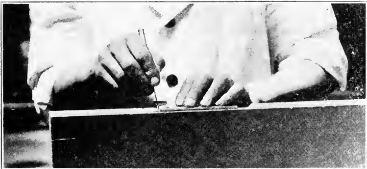
FIG. 449. MARKING HINGE LENGTH.
